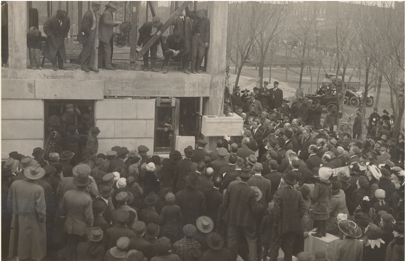
The cornerstone laying masonic ceremony, over the the construction of the Noble County Courthouse.
